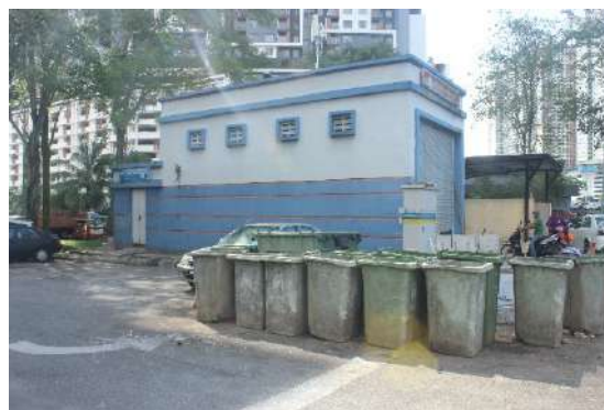
Figure 9. Bins outside of refuse chamber at PPR Seri Semarak
